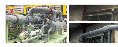
Ohio Valley Industrial Services manufactures a complete line of removable-reusable insulation jackets to meet most industrial, commercial and laboratory insulating requirements. HotCaps<sup>™</sup> are the cost effective way to insulate valves, flanges, expansion joints, and other components, providing the user with the energy savings associated with permanent insulation and the flexibility of reusing the cover.
