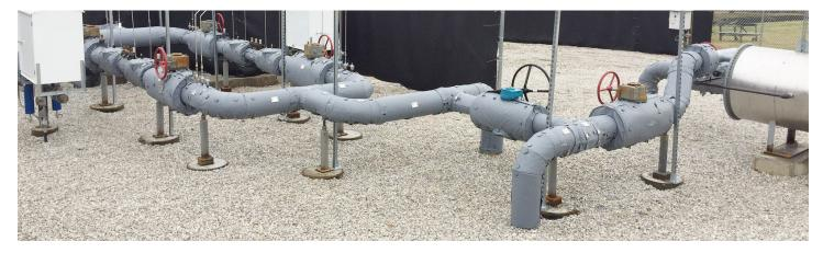
SoundCaps<sup>™</sup> by HotCaps<sup>™</sup> are a direct solution to sound control for any application. They are custom designed around your 2D drawing, 3D model, or already existing system to reduce sound directly at its source. These blankets are completely removable, reusable, and constructed using the highest quality materials for both indoor and outdoor use. SoundCaps<sup>™</sup> are designed to handle temperatures ranging from cryogenics to +2000F.
